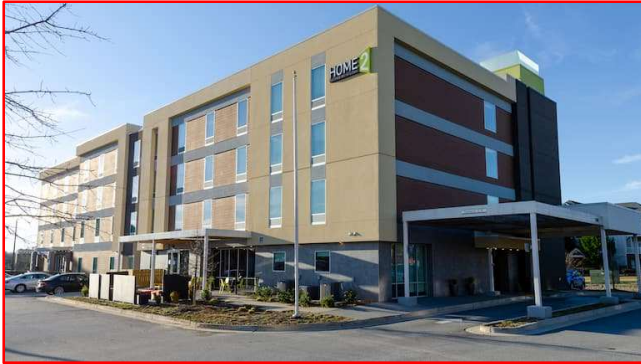
Home2 Suites by Hilton Atlanta Airport West Stop #1
