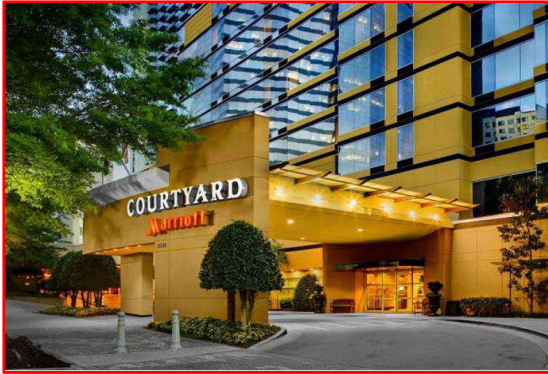
Courtyard Marriott Atlanta - Buckhead Stop #1
